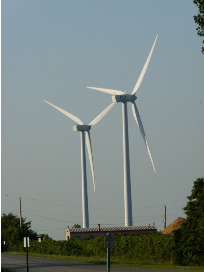
Figure 1: A pair of 1.8 MW wind turbines in Bowling Green, Ohio (photo by E. Nordman). These turbines are part of a four-turbine, 7.2 MW wind farm at the Wood County landfill.
