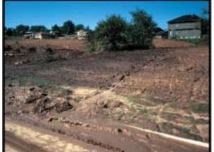
Sediment is seen in the street because measures were not taken to protect the soil from erosion during development. Photo courtesy of USDA-NRCS
