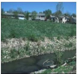
• Consult a professional landscaper or architect for solutions to control erosion and stabilize streambanks and shorelines. **Riprap** (piles of stone, rock, or broken concrete) is one stabilization technique for property next to surface water. Caution in the use of riprap is recommended in that it can often lead to impacts on adjacent property.
