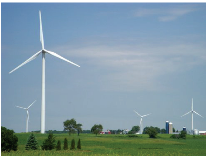
Figure 2a. Wind farm in Wisconsin with 86 turbines each at 1.5 MW capacity (Forward Wind Energy Center, 2009). (Dept of Energy – NREL)
