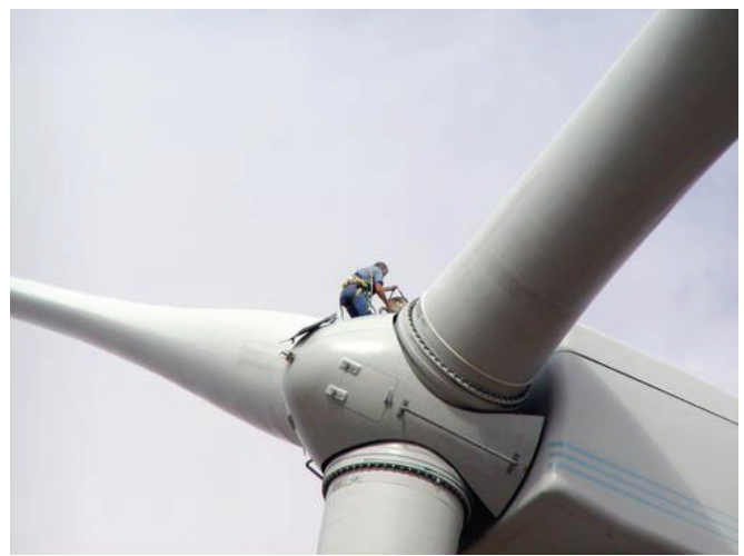
2b. Researcher entering the hub of a 1.5 MW wind turbine in Texas (GE Wind, TX, 2002). (Dept of Energy – NREL)
