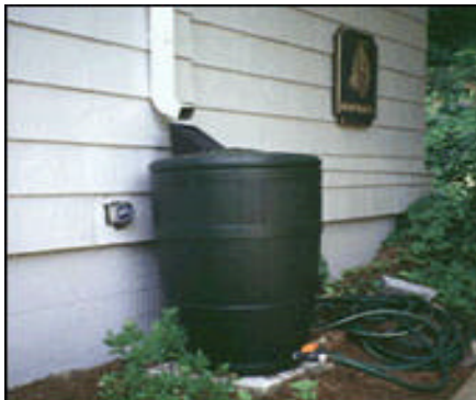
Rain barrels can be used to retain stormwater on site. Rain barrels provide a source of chemically untreated water for plants and compost while diverting water from uncontrolled dumping into storm drains.
