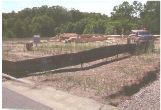
For sedimentation control, silt fences must be installed properly. The silt fence above is improperly installed because it is not trenched into the ground.
