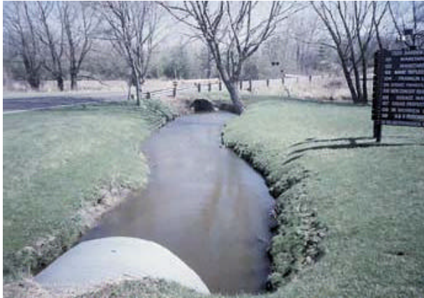
The status of existing infrastructure is an important factor in establishing a plan. To identify existing infrastructure, verify the location and type of culvert and upstream and downstream culvert size.
