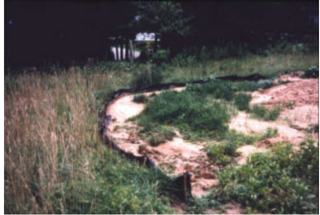
Utilizing a series of Best Management Practices is important to minimize runoff. In the picture above, a silt fence and buffer strip are used together to minimize the amount of sediment being swept off the site during a rain event.
