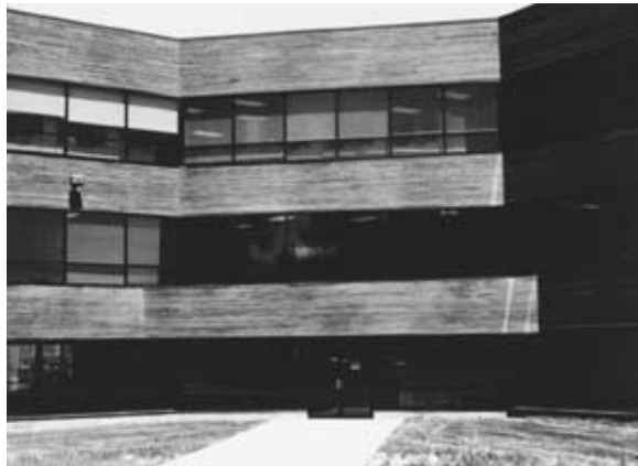
Figure 6: Far View of Modern Building Low in Visual Richness but With a Visible Entrance
