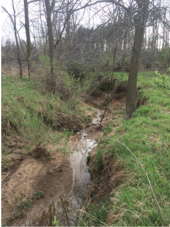
Figure 3.14. Severe incising and bank erosion observed in Walker Avenue Ditch (subbasin B11) of the Indian Mill Creek watershed, April 2017.
