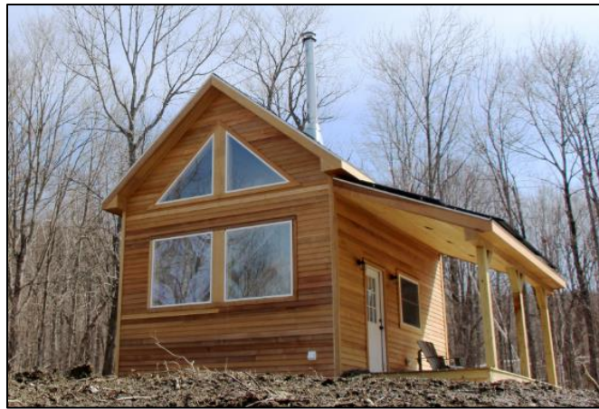
Figure 4: Example of a Tiny House Built on a Foundation [4]
